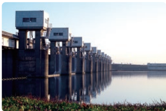
For River Water Level Control
