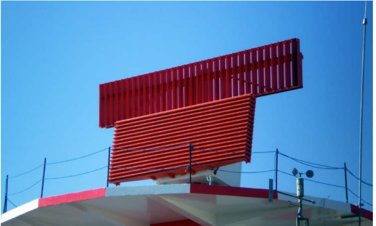
3D PSR &amp; MSSR Antennas
