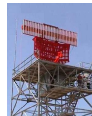
Figure 14: ASR-12, a typically Air Surveillance Radar
