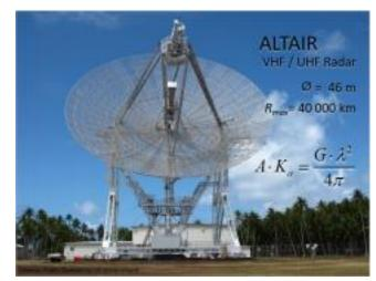
equation with the antenna gain: For a desired (constant) antenna gain, the size of the antenna is proportional to the wavelength. That means: if the antenna gain is the same, the necessary geometrical extension of the antenna will also be larger with a larger wavelength! The picture shows a VHF/UHF radar with a parabolic reflector with a diameter of 46 m.
