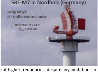
radars with higher accuracy requirements operate at higher frequencies, despite any limitations in range.
